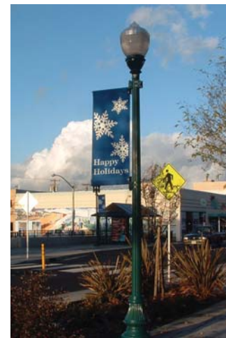
Street Light Head - HADCO R33BBNN1JGBG150SE Pole + Base - VISCO B17-F/12-3"x3" Green Powdercoat
